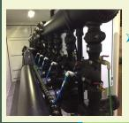
Tubing color coded to industry standards and spiral wrapped for protection.
