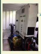
Control panel positioned with pressure gauges installed at point of use.
